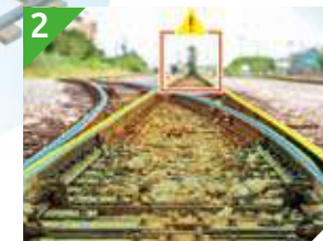
Track obstacle/ intrusion inspection
